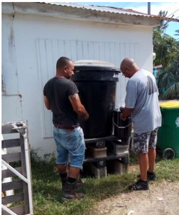
Above: placing 150 gallon drum on pallets & installing 2 taps
